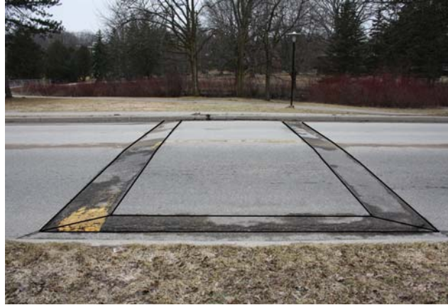
Figure 44: The first bump on Ring Road.
